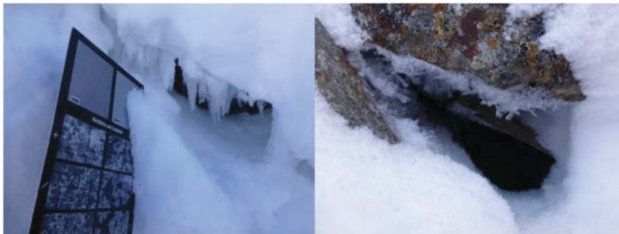
Fig. 9. Cavity hoar in joint apertures under a thick snowpack in mid-winter in the North facing rock wall at Gemsstock. The snow crystal card on the left is 20 cm long. Photographs: M. Phillips.
