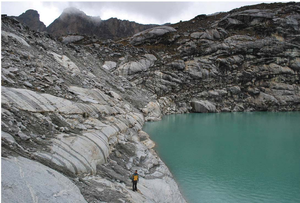
Figure 7. Exposed adverse slope of the Laguna 513 bedrock overdeepening in the Cordillera Blanca (cf. Figures 1 and 4). The level of the lake had been artificially lowered by 20 m with the construction of tunnels in the bedrock threshold for hazard prevention (Carey et al. , 2012); the original overflow was about 20 m above the person in the foreground. Note the absence of a deeply incised rock channel in the smoothly polished 'riegel'. Photograph: C. Giraldez 2012. This figure is available in colour online at wileyonlinelibrary.com/journal/esp
