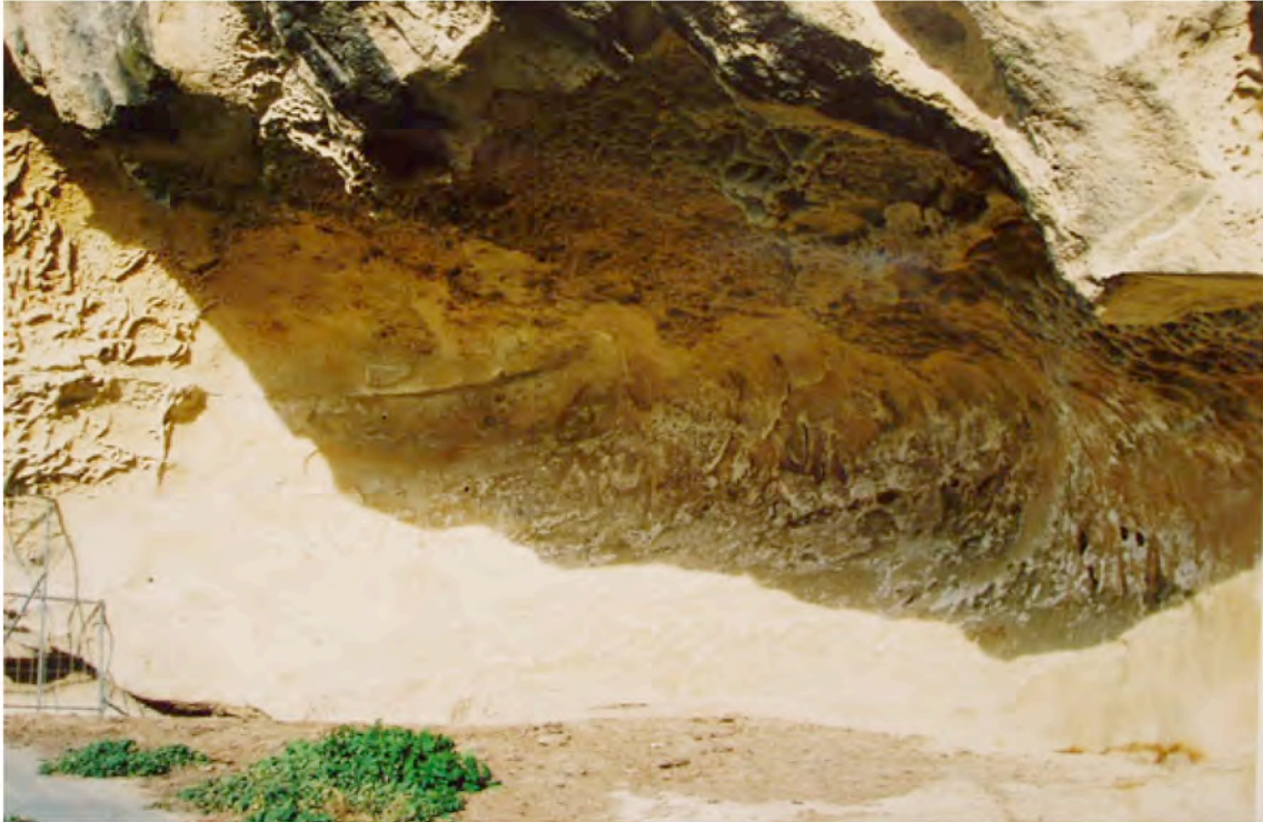
M1" (29.06.05): the salts and algae are clearly visible in the shaded area. There is not so much stock excrement on the ground, but there are brown lines at the bottom of the alcove presumably from this source. The graffiti are not as visible given the light condition, but a large white ONLY can be read in the sunny area.
