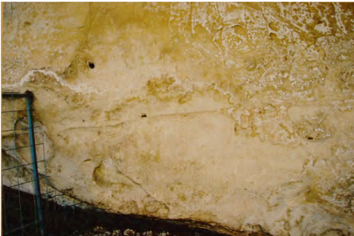
M1' (28.06.2005) : fig 96-97-98 are still visible, but very faint. The erosion is progressing, and there are a lot more salts in the upper part of the alcove and towards the left. There is also a significant quantity of green moss ( or algae?). The hole seems stable as well as the exfoliation. The heart-shaped area of salt is still there, same shape, and the engraved M as well, showing that very little erosion has occurred there during the last 10 years.
