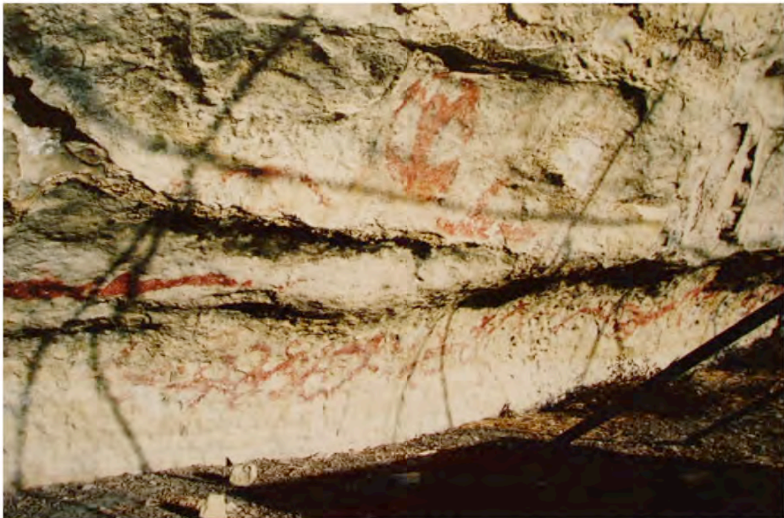
M1' (28.06.2005) : The ground is the same, the plant is not there but there is another one nearby. Absolutely no change to describe, except for some changes in the disintegrated area under fig 61a and salts in the eroded area on the left. It must be noted that a flake from 61c has been lost during the photographic survey of 1992-3, because it was present on photo BJA 61b and is now lacking on photo BJA 59-62. The rock is still very dark underneath the second overhang.
