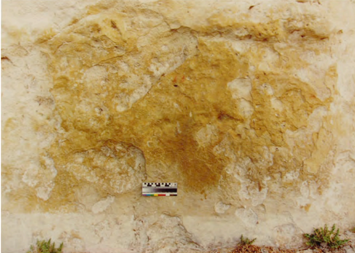
Photo by B.J.A. (summer 1992-3): 4a is clearly visible, on a yellow regular surface. There are some bird droppings in some areas. An area of exfoliation is situated to the right of the motif. There is a small amount of vegetation on the ground (no grass).
