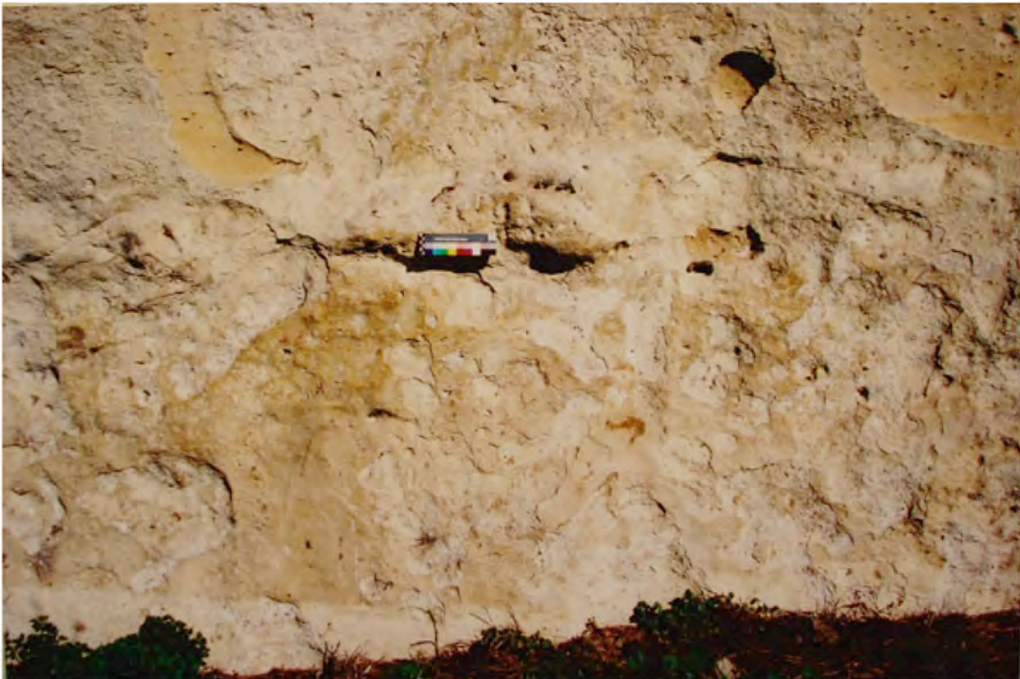
M1 (05.04.2005): Fig 4a, 4b and 4c still visible. No noticeable extension of exfoliation. Bird droppings washed away but new ones have appeared. Vegetation changed in species but not in quantity or volume. There is a dark stain under fig. 4b. Surface clearer than before, perhaps due to wetting.
