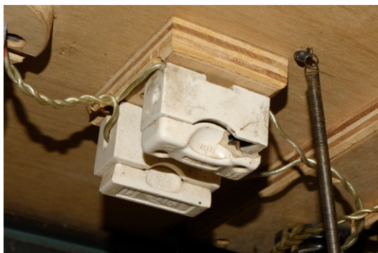
Fig. 122: Fuses with one of the lids broken
