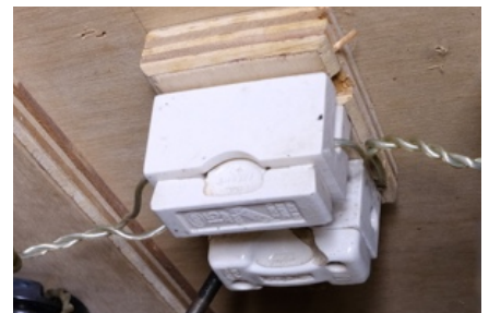
Fig. 71: The fuses fixed on the ceiling of the upper compartment
