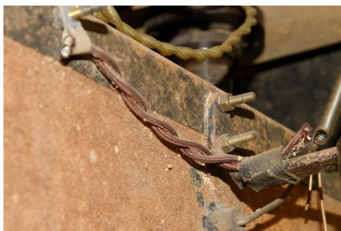
Fig. 124: Old wire that has been cut, near the lamp 5 on the back of the display panel
