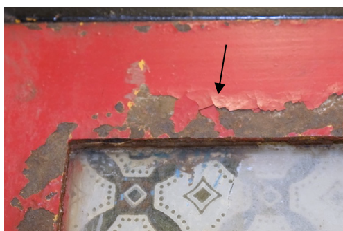
Fig. 139: Lifting of the paint layer on the upper right panel before treatment
