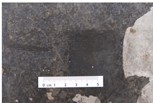
Fig. 141: Zone of the roof after the smoke sponge cleaning
