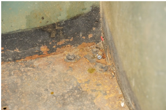
Fig. 108: Unattached bolts found on the base of the lower compartment
