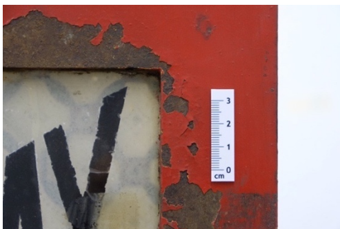
Fig. 94: Lifting of the red paint layer near the losses
