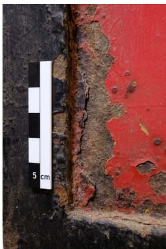
Fig. 98: Delamination with loss of the paint layer
