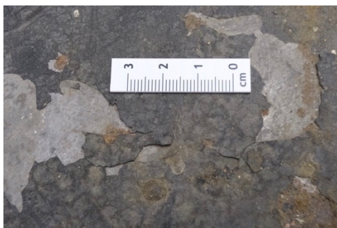
Fig. 92: Dust on the roof, with the lifting of the paint layer and presence of corrosion spots
