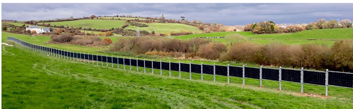
Figure 47 : Exemple barrière photovoltaïque bifaciale ( https://next2sun.de/wp-content/uploads/2020/01/Irland_waterford.jpg )
